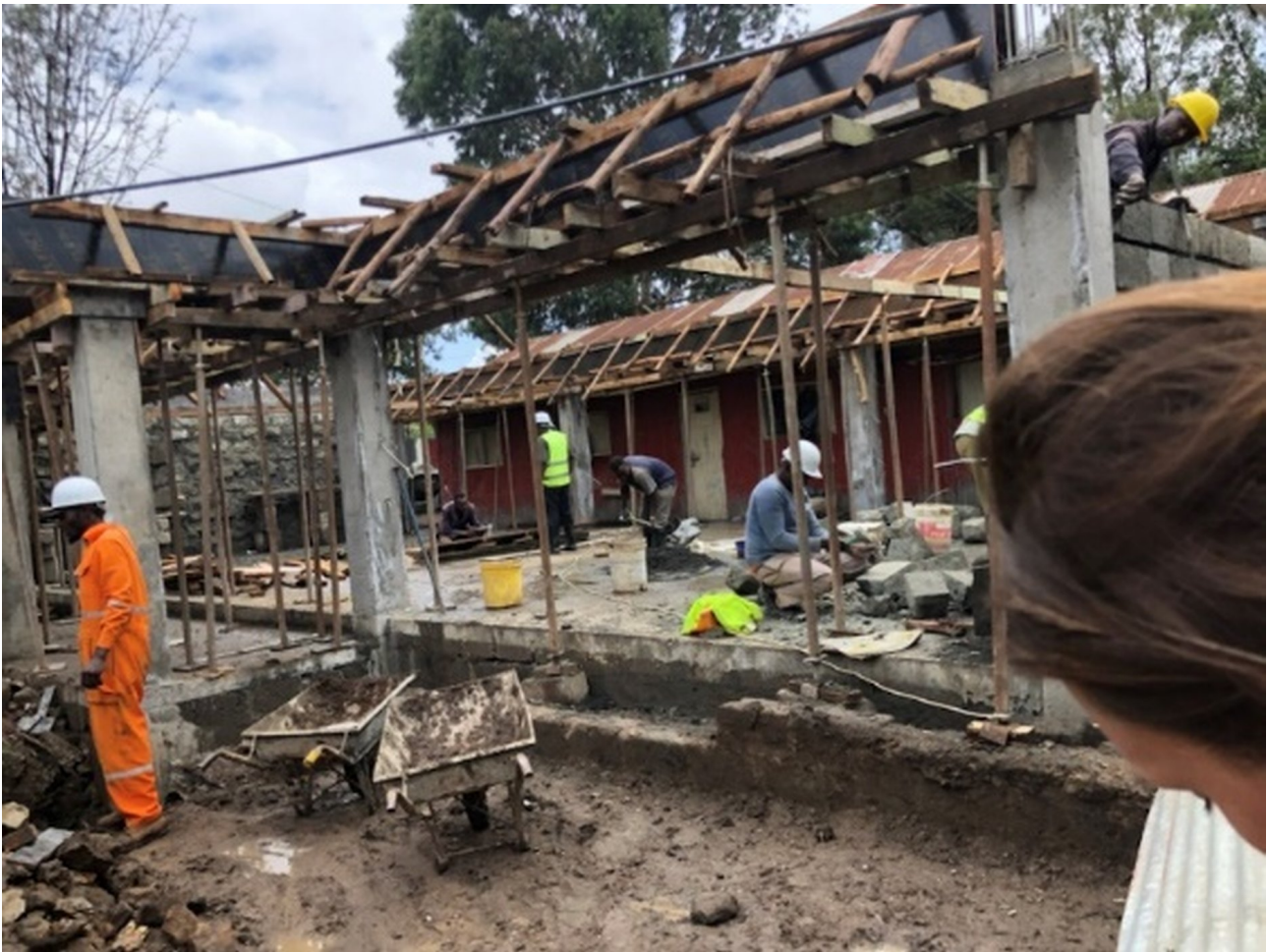
The new dining room in the Mukuru Promotion Centre under construction.
