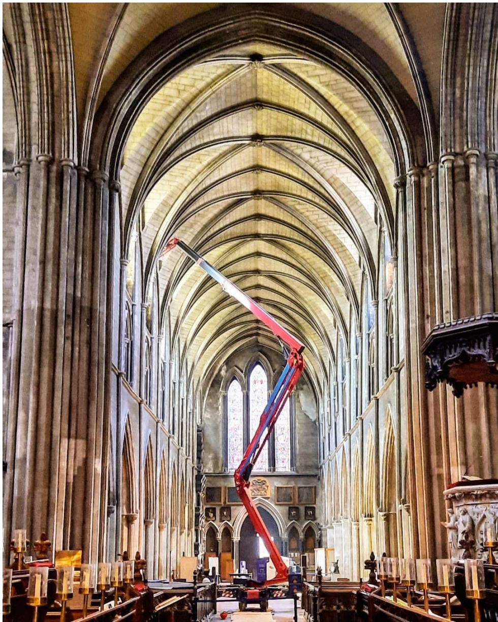
Image of the day - St Patrick's Cathedral Dublin, Celestory windows restored
