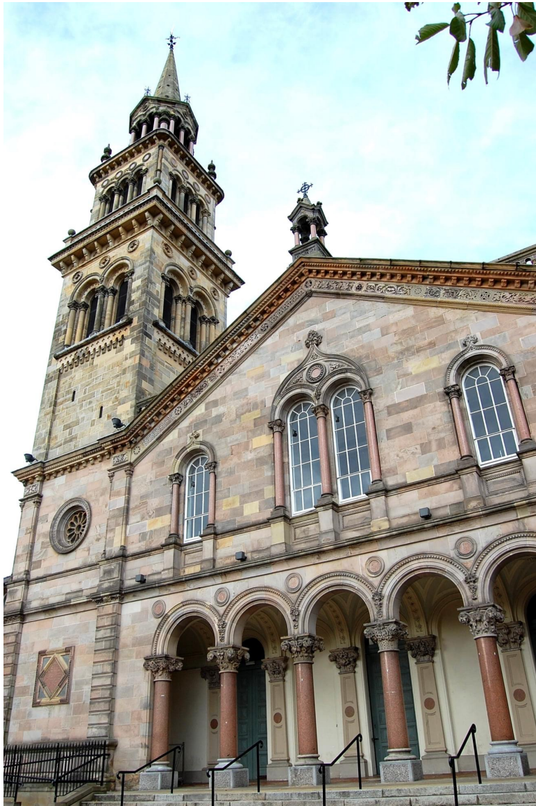
Image of the day - the former Elmwood Presbyterian Church
