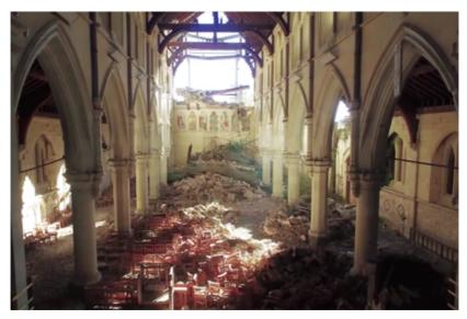
Still image from a video produced by a drone camera inside New Zealand's Christchurch Cathedral showing damaged caused by the February 2011 earthquake.
